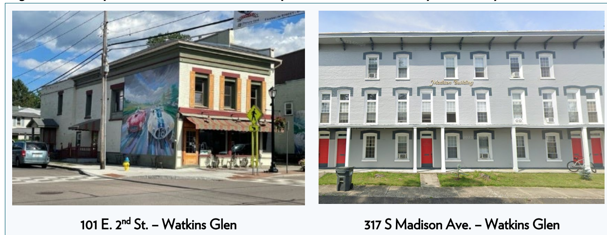
Figure 33: Sample of Available Individual Apartment Units in Schuyler County
